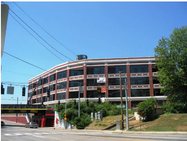
Condominiums in former Ford Motor Co. Plant, Louisville
