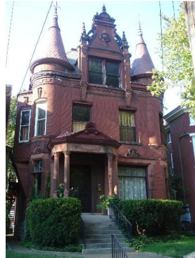
Residential building, Louisville
