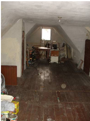
Attic Space Before Renovation
