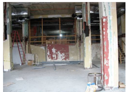
1st floor Rehabilitation work
