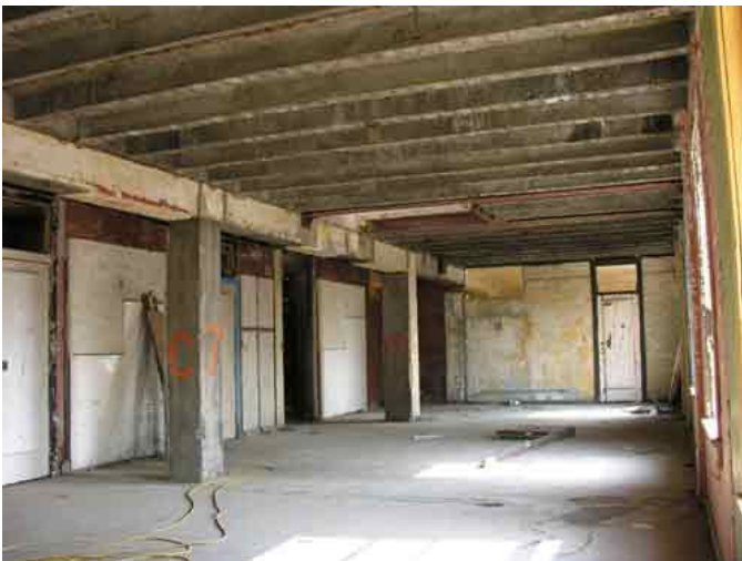
Renovation of Hotel rooms into Lofts, Henry Clay, Louisville
