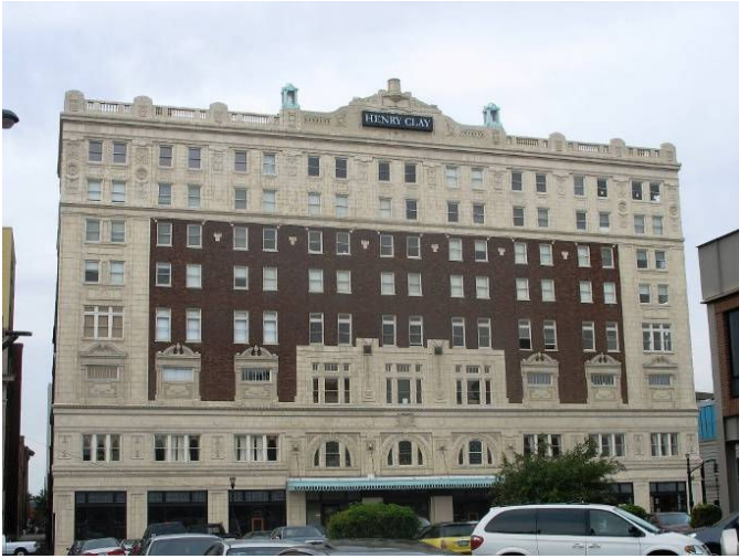
Henry Clay post-restoration
