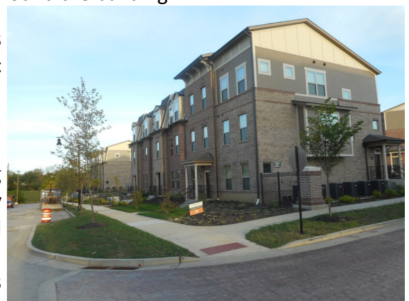
ADA compliant, tree-lined sidewalks provide continuous connectivity in the River's Edge community.
